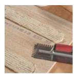
Panels can be adhered to concrete, drywall and plaster with Titebond® GREENchoice Acoustical Ceiling Tile Adhesive. Follow adhesive manufacturer's instructions for application and usage.
