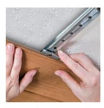
WoodHaven<sup>™</sup> plank installation using Easy Up® tracks and clips
