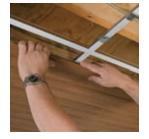
Position planks; slide and secure clips
