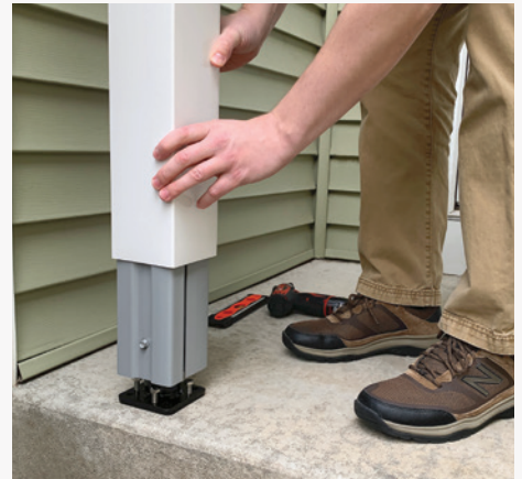
Attach fillers and place sleeve over post.
