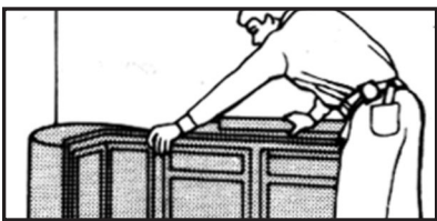
Start base cabinets in corner
