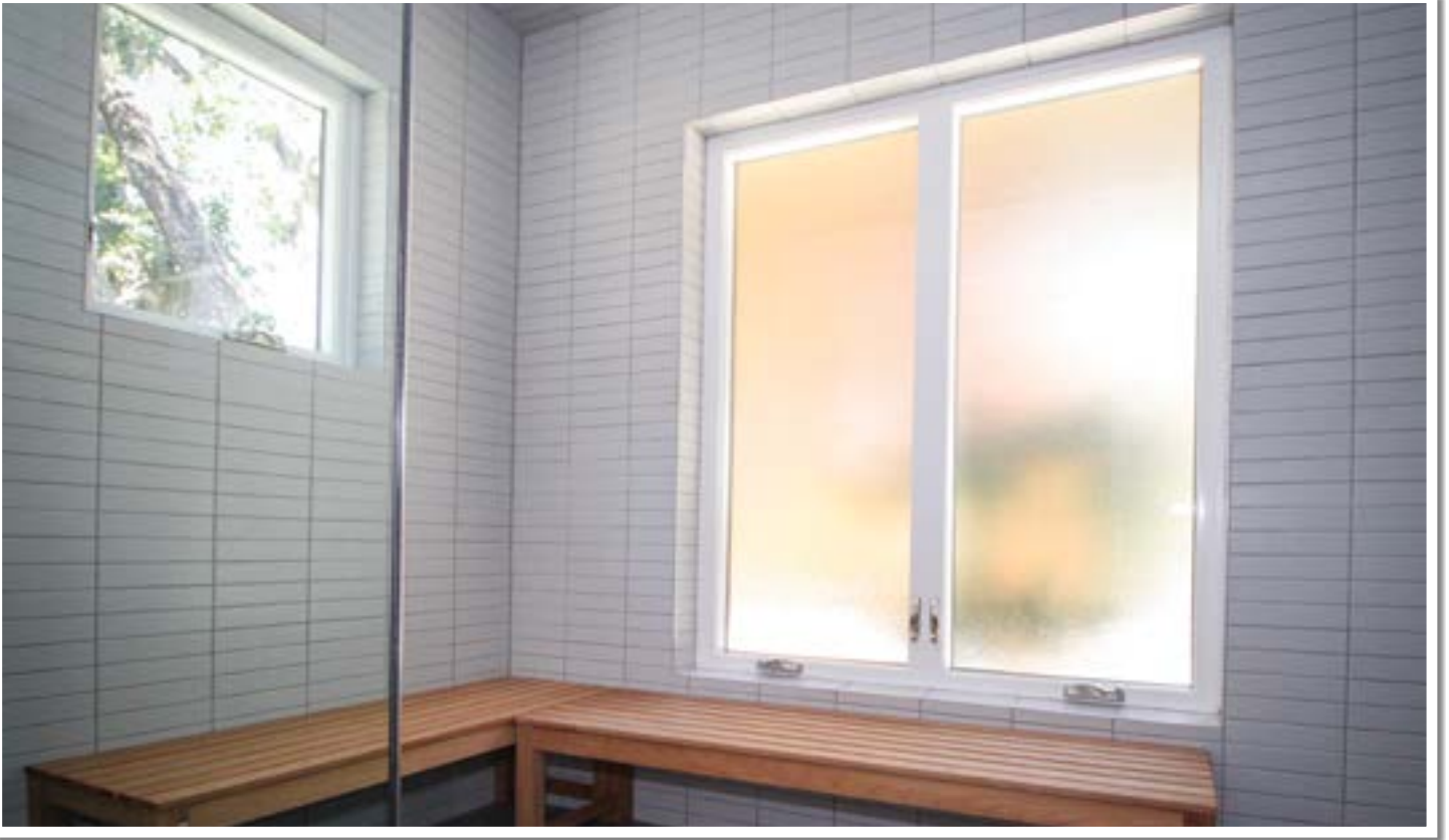
Above: Obscure glass provides privacy and lets in natural light, making it the ideal choice for this steamroom. A twin casement with stainless steel hardware.
