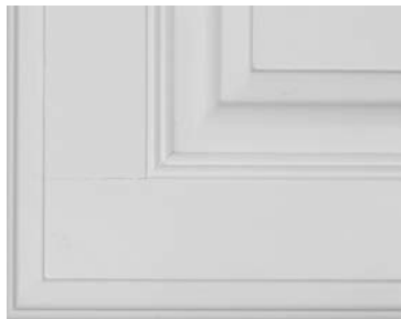
Example of front joint separation
